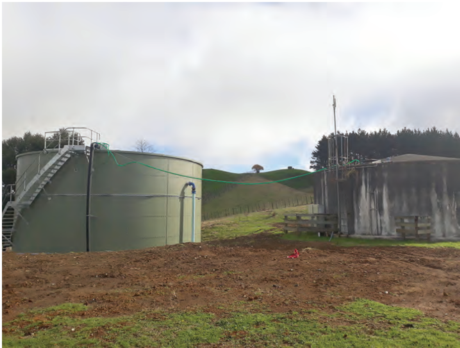
NEW PIOPIO WATER RESERVOIR (LEFT) AND OLD (RIGHT).
