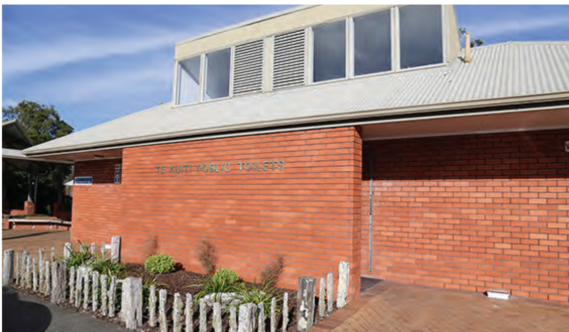
RORA STREET PUBLIC TOILETS
