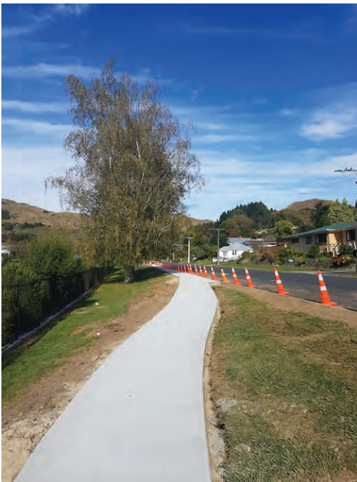
KING STREET WEST FOOTPATH TO PUKENUI PRIMARY SCHOOL
