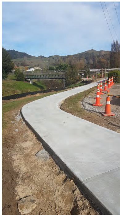
ESPLANADE FOOTPATH ADJACENT TO TE KUITI BOWLING CLUB
