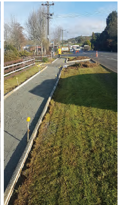
CONSTRUCTION OF NEW FOOTPATH UNDERWAY -MOA STREET PIOPIO
